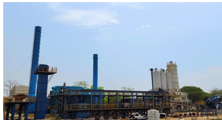
Ash to Sand Facility at NTPC Sipat
